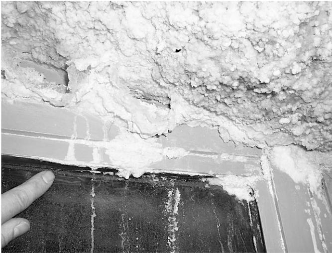
**Figure 5.** Detail of the frame of the glass door. Aluminum sulfate crystals are growing on outer side on aluminum frame, along rubber joints. Outside temperature is 24 °C, inside temperature is 37 °C; humidity at saturation produces condensation on the glass.
